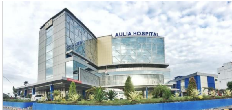
Gambar 5.1 Aulia Hospital Pekanbaru
