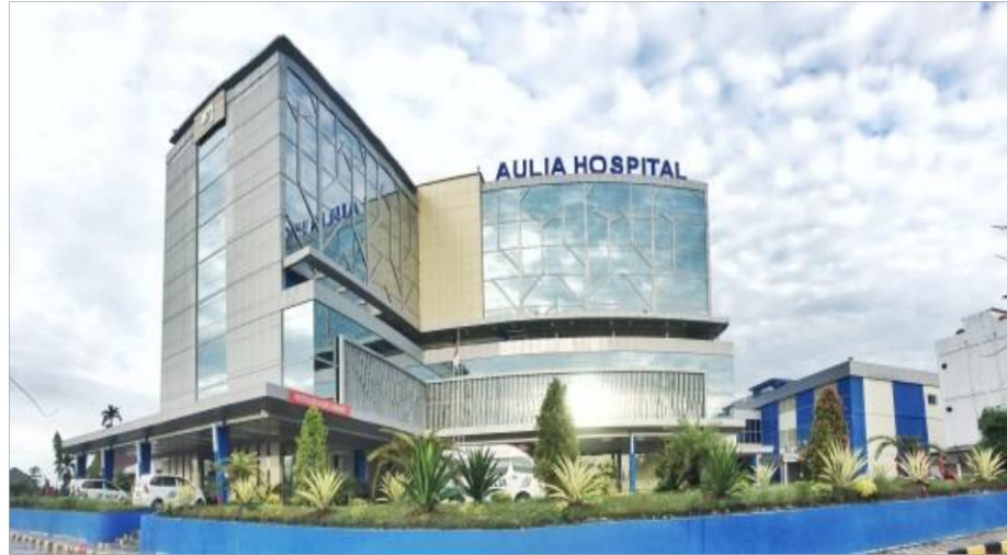
Gambar 4.1 Aulia Hospital Pekanbaru
